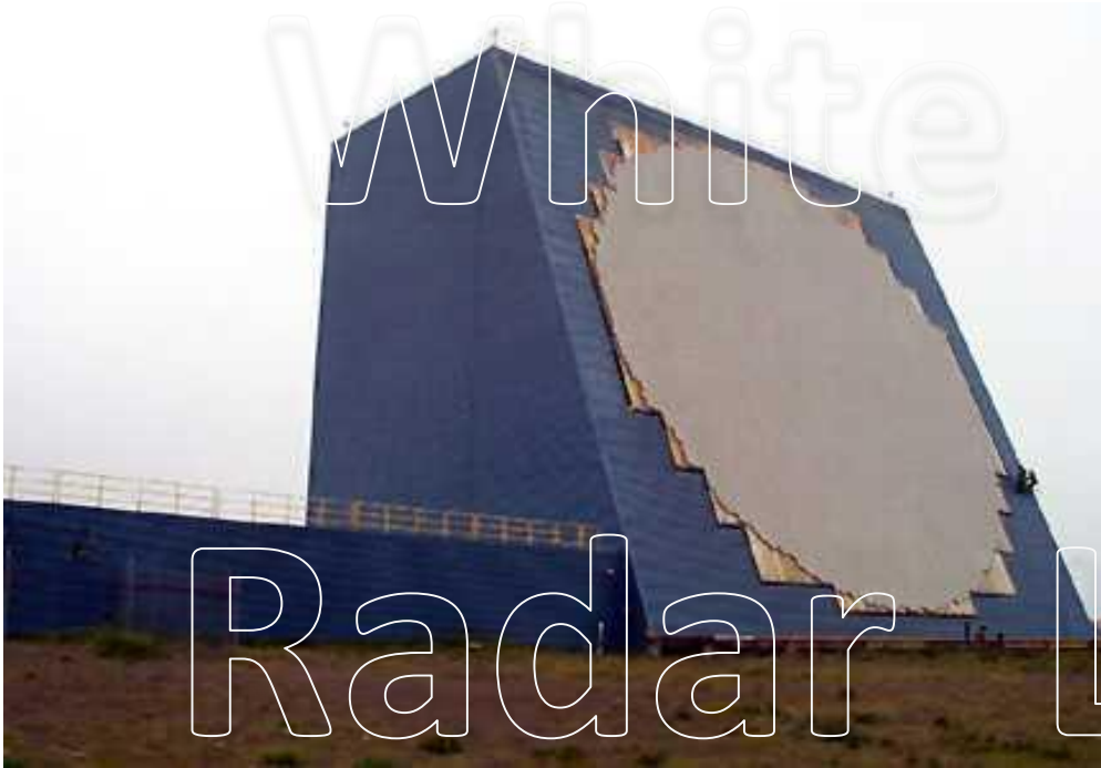
ICBM Detection Radar 400 - 500 MHz, 30 m high, 3000 km range
